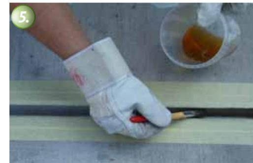
Absorbent substrates must be primed with KÖSTER FS Primer twice. Non-absorbent substrates are primed once.
