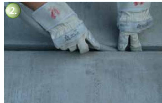
To avoid damages to the Joint Sealant caused by movement in multiple directions, the Joint Sealant should only bond to two joint flanks. For this reason a backing is installed for example with quartz sand or a foam PE backing rod. This eliminates the possibility of adhesion to three flanks.
