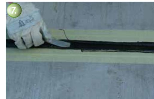
The Joint Sealant is smoothed, for example with a spackle. The tape should be removed before the Joint Sealant has hardened.
