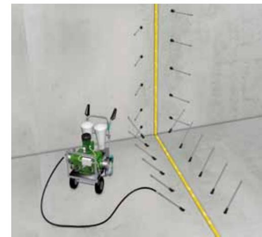
Waterproofing joints that are moist or even have water flowing through them are a special challenge, as many waterproofing sealants will not bond to wet or even moist substrates.
