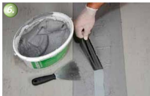
For optical reasons the black tape in the center of the KÖSTER Joint Tape can be covered with KÖSTER KB-Pox® Adhesive and removed before the Adhesive begins to cure.
