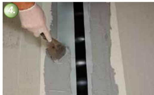
The KÖSTER Joint Tape is embedded into the fresh adhesive. Immediately thereafter the second layer of adhesive is applied.
