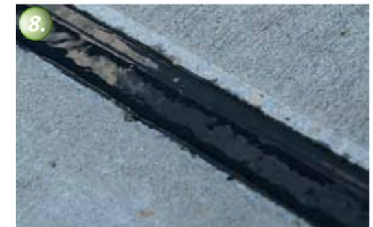
KÖSTER Joint Sealant FS-H in its cured state.
