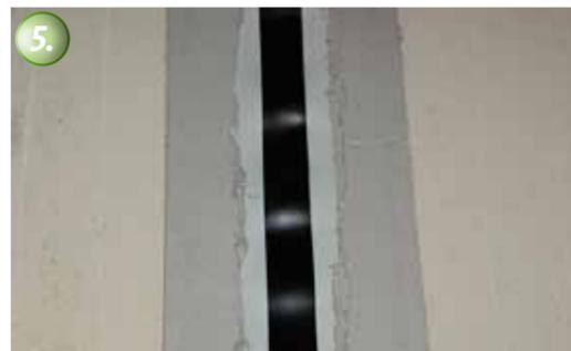
The masking tape on both sides of the KÖSTER Joint Tape must be removed before the KÖSTER KB-Pox® Adhesive has begun to cure, so that a clean boundary results. The KÖSTER KB-Pox® Adhesive must cure for 24 hours.
