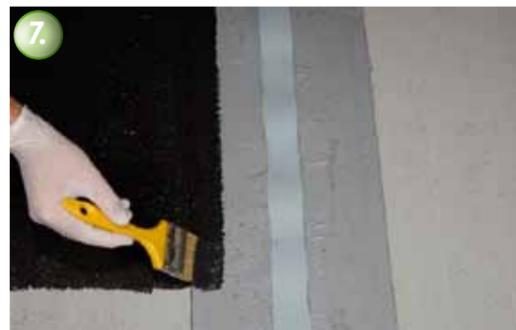
After the KÖSTER KB-Pox® Adhesive has cured for 24 hours the area waterproofing can be applied overlapping the KÖSTER Joint Tape.
