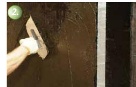
An area waterproofing such as KÖSTER Deuxan® 2C is easily overlapped onto the KÖSTER Special Joint Tape.
