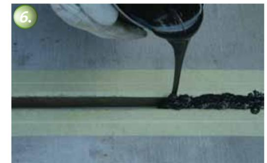
The joint is filled approximately 2 hours after applying the KÖSTER FS Primer.
