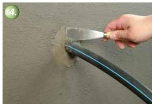
The pipe penetration is now permanently waterproofed.
