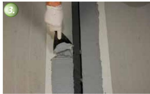
The two components of the KÖSTER KB-Pox® Adhesive are mixed according to the Technical Guideline until a homogenous grey color is reached. The Adhesive is then spread onto both sides of the joint 2-3 mm thick.
