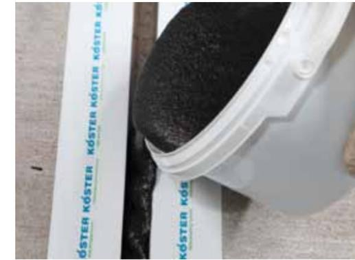
KÖSTER PU Joint Sealant is chemically stable when hardened and highly resistant to organic and inorganic acids, alkalis, and will not rot.
