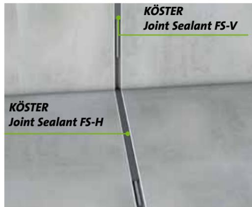
A commonly used method for waterproofing joints is to fill them with an elastic material. KÖSTER Joint Sealant FS-H is a self leveling, rubbery-elastic sealing compound with high chemical resistance and is therefore the ideal material to waterproof horizontal joints in heavy construction, in foundations, waste water treatment plants, garages, tunnels, etc. KÖSTER Joint Sealant FS-V has a putty-like consistency for vertical and horizontal joint waterproofing.
