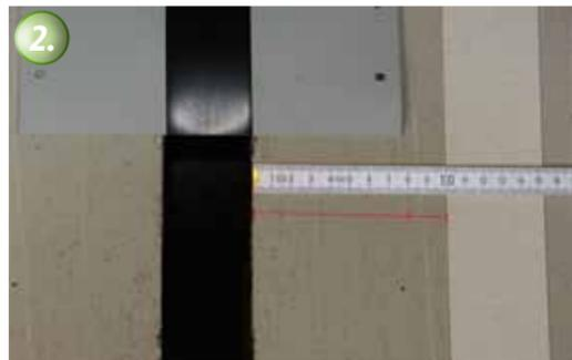
KÖSTER Joint Tape 20 is embedded into the adhesive at least 4 cm on each side (the KÖSTER Joint Tape 30 at least 5 cm). The adhesive is applied 2 cm farther onto the substrate.
