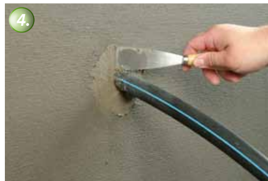
The pipe penetration is now permanently waterproofed.
