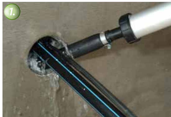
KÖSTER KB-Flex 200 can even be used under flowing and pressurized water.
