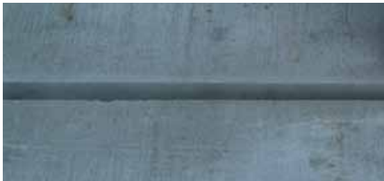
Cleaned joint flanks
