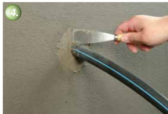
The pipe penetration is now permanently waterproofed.
