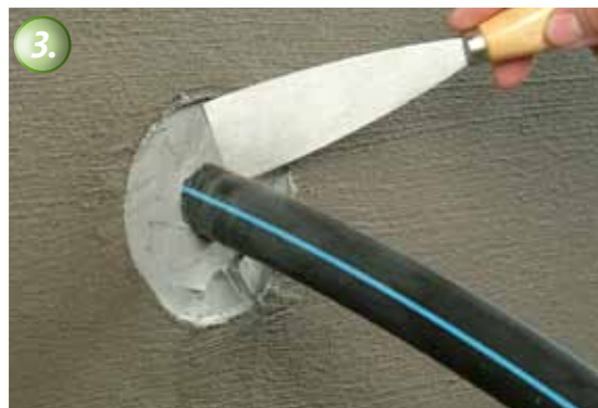
To protect the waterproofing the area is smoothed and protected with KÖSTER KB-Fix 5.
