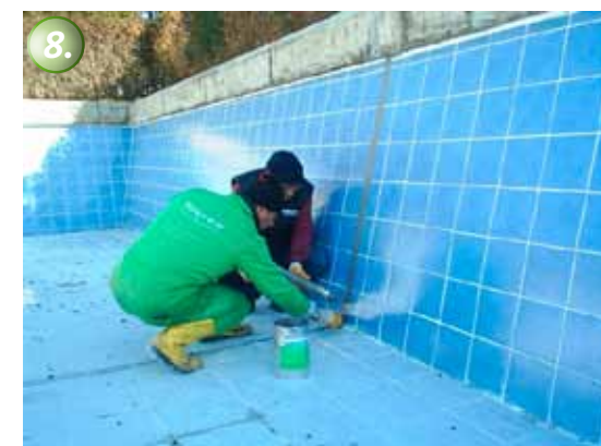
8. The horizontal joints are waterproofed with KÖSTER Joint Sealant FS-H. The vertical joints were waterproofed with the putty-like KÖSTER Joint Sealant FS-V.
