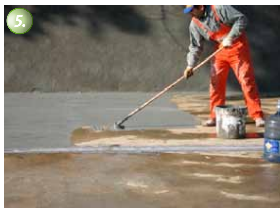
5. The area waterproofing is done with KÖSTER NB 1 Grey. KÖSTER NB 1 Grey is a mineral based waterproofing against ground moisture, non-pressurized and pressurized water. KÖSTER NB 1 Grey is resistant to positive and negative side water pressure.
