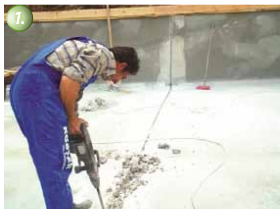
1. The debris and remnants of the concreting work are removed.
