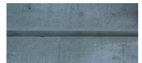
Cleaned joint flanks
