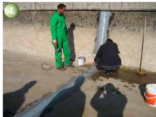
4. Connections are made with a hot air welding gun; seams should overlap at least 2 cm.
