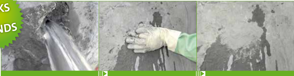
An active leakage is sealed instantly after applying KÖSTER KD 2 Blitz.
