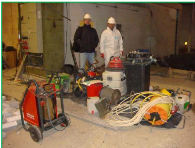
Pic. 7: KÖSTER ORS Products / OERTZEN Washing & Vacuuming Machinery
