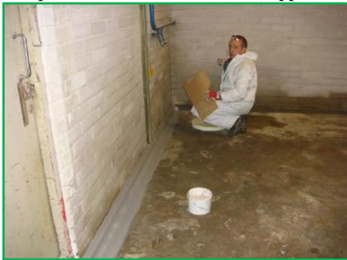
Pic. 17: Application of the oil resistant coating KÖSTER ORS C...
