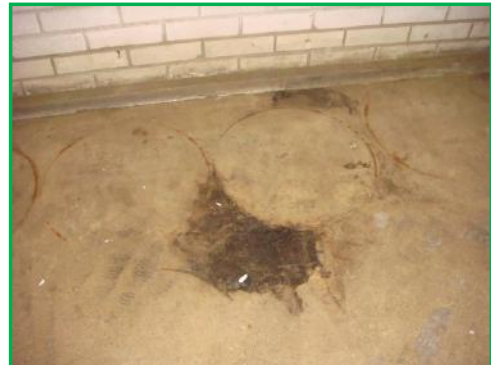
Pic. 11: Floor after washing with the Turbo Jet and after vacuuming
