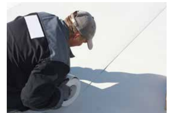
The membrane is positioned and then welded.
