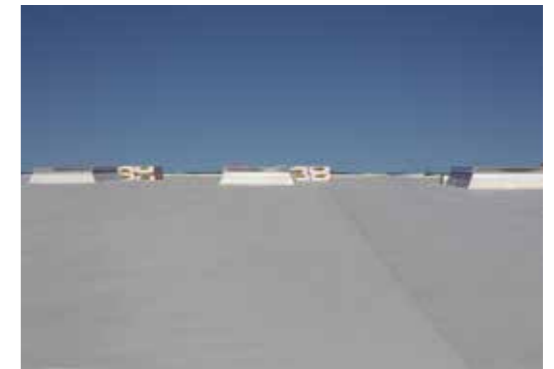
KÖSTER TPO Membranes are connected to individual SHEV-flaps with KÖSTER Contact Adhesive.
