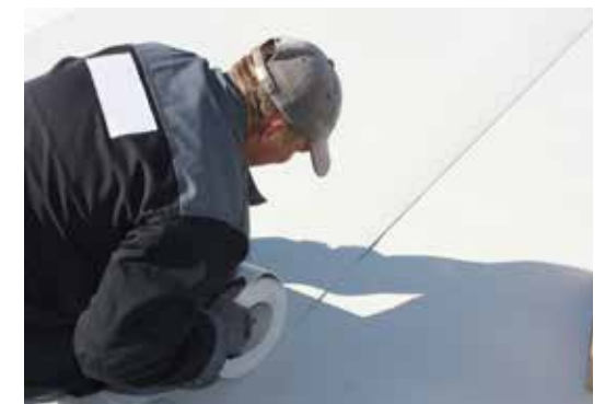
The membrane is positioned and then welded.
