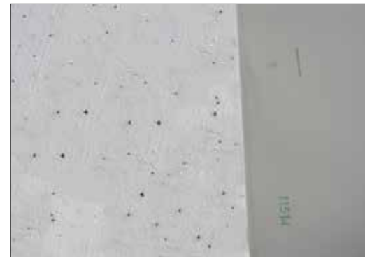
Direct installation over EPS insulation
